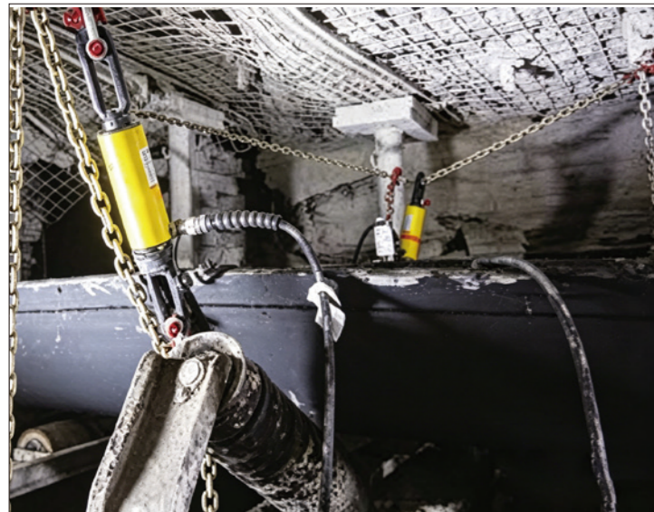
▼ Lifting mining conveyor belt using pull cylinders for bearing maintenance.
