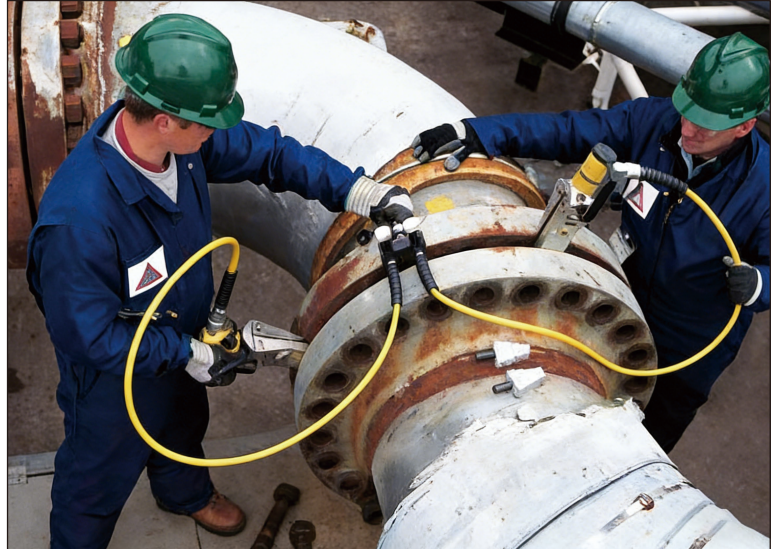
Two FSH14 flange spreaders used simultaneously with a RIVERLAKE hand pump, Hose 1 and AM21 manifold block.
