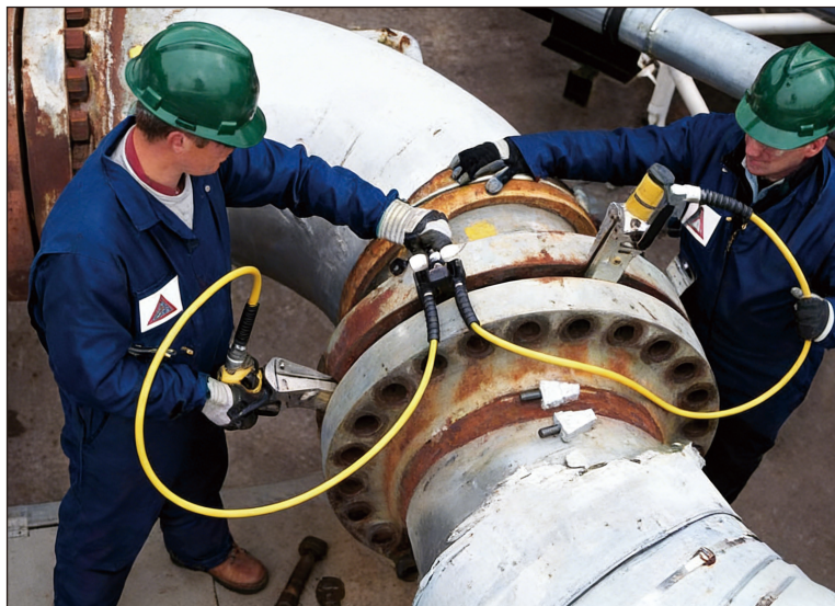
Two FSH14 flange spreaders used simultaneously with a RIVERLAKE hand pump, Hose 1 and AM21 manifold block.
